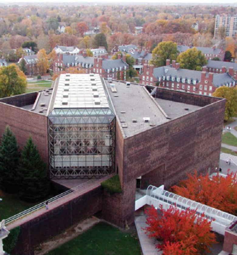
View from the Bell Tower
